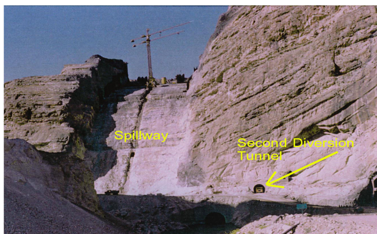
Fig.5. A photo of the second diversion tunnel in the left abutment.
