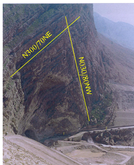
Fig.8. Several joint sets cut the Asmari limestone at the site. The rock mass is cut by two major sets of joints. One major joint set strikes 030 and dips 80 degree NW. The other major joints set strike 300 degree and dips 70 degree NE.
