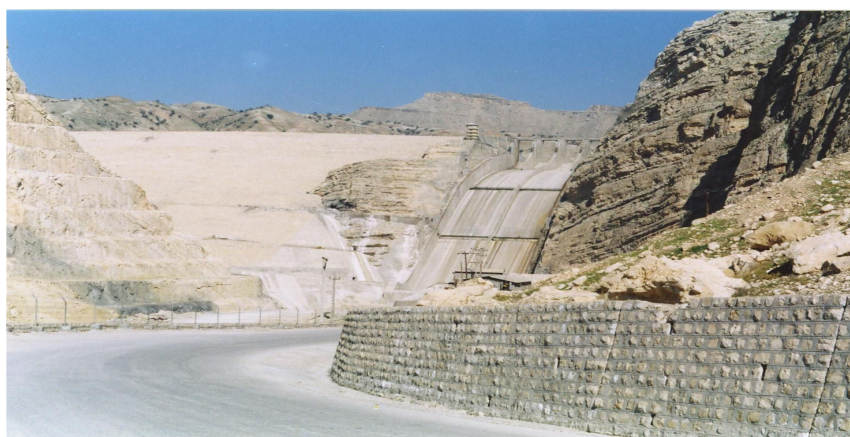
Fig.2. A photo of Marum dam (downstream).
