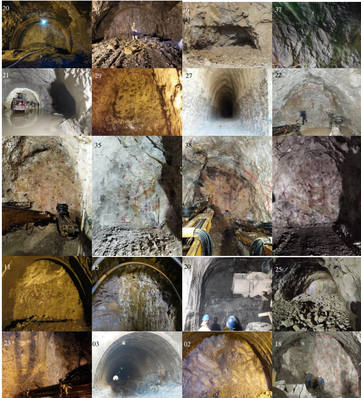
Fig. 2. Images of some of the studied tunnels (the number of each image corresponds to the tunnel number in Table 1).
