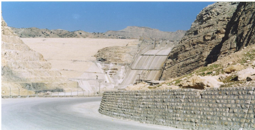
Fig.2. A photo of Marum dam (downstream).
